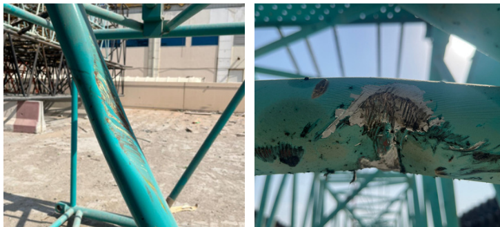
Bended and Dented Pipe
